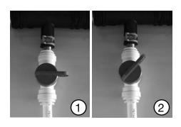
The flow control and thus the efficiency of the two water circuits (living room/bedroom) can be regulated by means of the shutoff valves.
